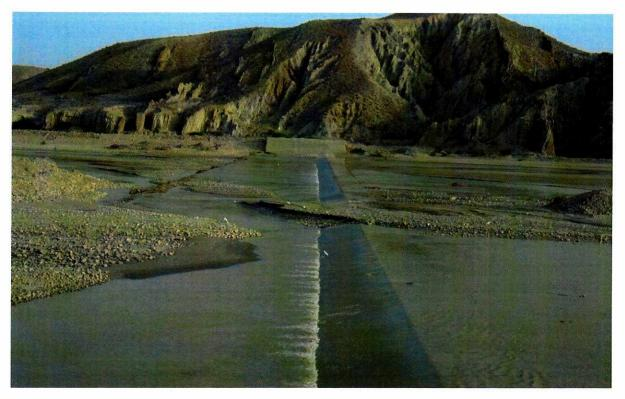
Jam- jat Wah Complex (Dispersion Structure) Constructed At Sanghar Hill Torrent
